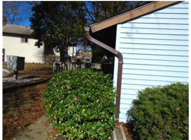
**Siding and Trim.** The buildings are clad in vinyl siding and trim. The overall condition of the siding is good. The siding is in the latter stage of normal service life and developing a comprehensive replacement program should be considered.
