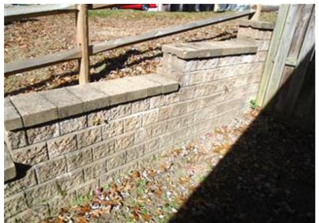
**Fencing.** The Association maintains a limited quantity of split rail fencing. The fencing is in good overall condition. The largest section is atop the segmented block retaining wall. This fence should be periodically inspected to ensure there are no issues, as this is a protective barrier fence.
