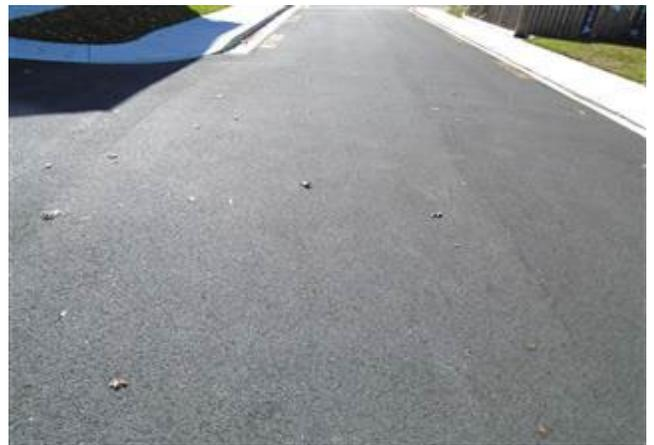
**Concrete Work.** The concrete work includes the community's curb, gutter, sidewalks, and lead walks. Usually, curb and gutter replacement should be performed when the asphalt pavement is overlaid. The association performed extensive replacement of curb, gutter, and sidewalks during the recent resurfacing of the roadways. The overall condition of the concrete work is in good condition. Some of the lead walks are displaying defects.
