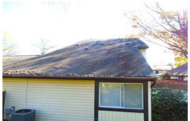
**Gutters and Downspouts.** The buildings have aluminum gutters and downspouts, there are 4' and 6" gutters and downspouts. The gutters and downspouts are in varying conditions. Future funding for replacement in conjunction with the roof shingles has been programmed in the analysis. Some downspouts have underground piping to direct outflow.
